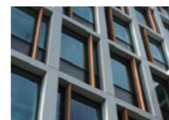
Facade design of utilizing a terra-cotta louver system
