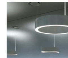
Arrangement of space using LED lighting
